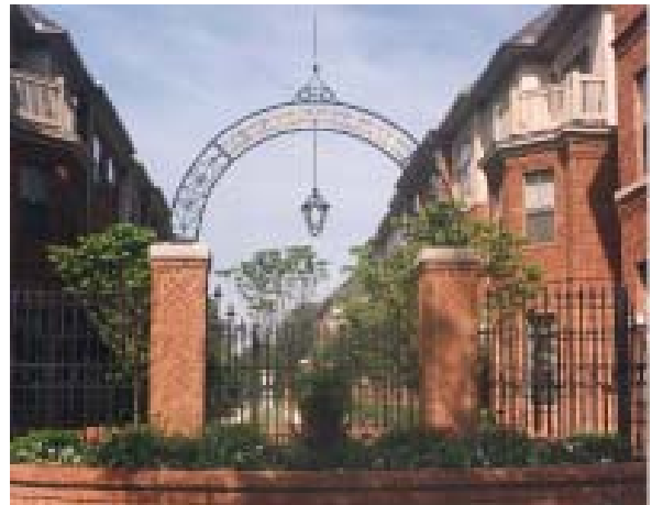
Victorian Gate is a new urban development surrounded by old neighborhoods.
